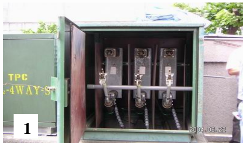
1. Cut off the high-pressure switch of Utilities Electric Co.
