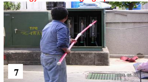
7. Connect and go to the high-pressure switch of Utilities Electric Co.
